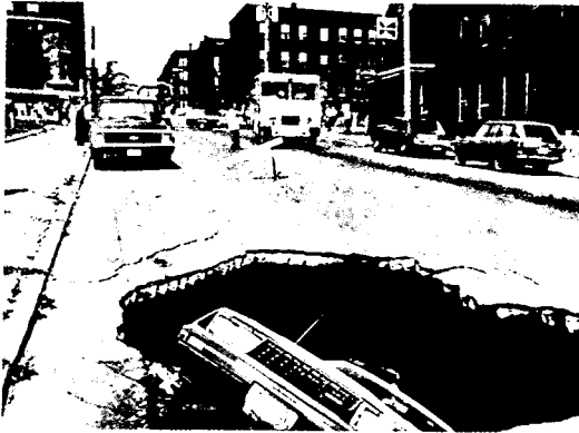
Undermining of roadways can occur without warning and lead to major disruptions.
